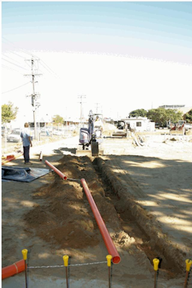
Site looking W – Installing the conduit under the slab that will contain the audio cables that run from the sound desk to the stage
