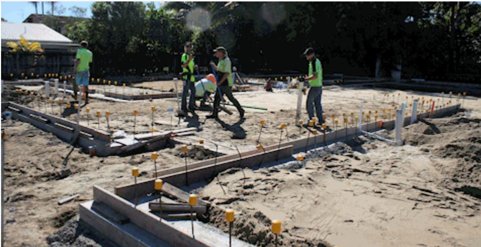
Site looking NE – Workers screening the sand on which the slab will be poured.
