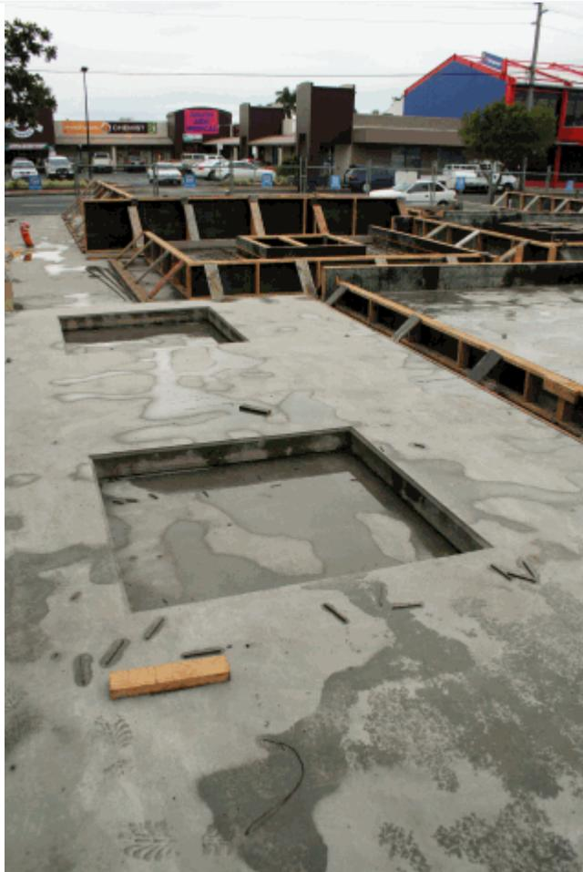
Site looking S – A completed panel with window spaces. This pan will actually be above the doorways that open onto the deck and kitchen area.
