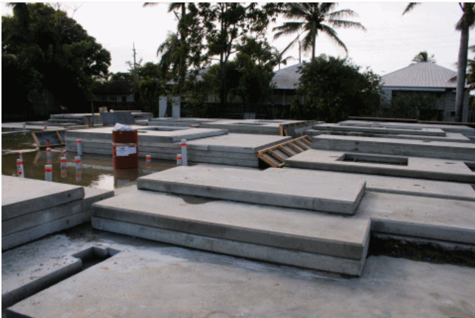
All of the panels, set up like tiles, ready to be lifted. Don't worry about the little water near the bathroom.
