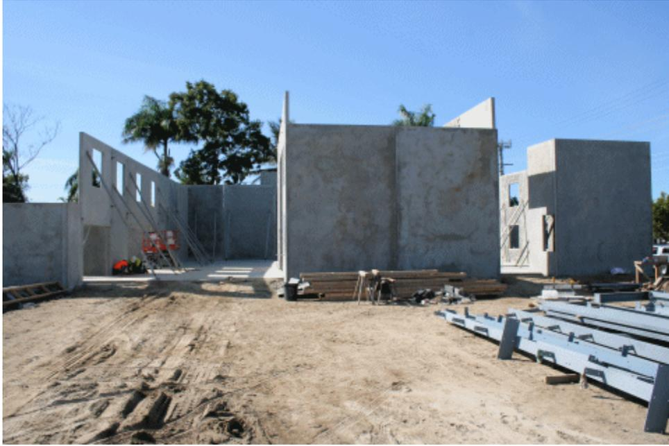
The front of the building. The main entrance is on the right. The open space to the left is where another entrance and the crèche will be. There are a small number of panels still to lift to complete this wall. Structural steel delivered on the right.
