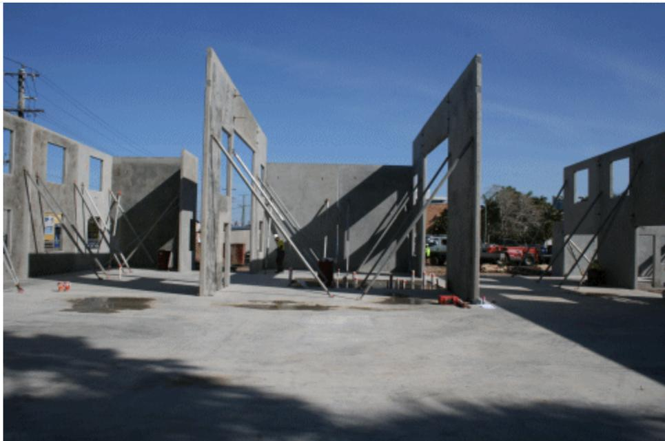
Standing from the front of the auditorium (stage) looking back. The two walls you see will be enclosed with concrete blocks from the left to the right of the photo.
