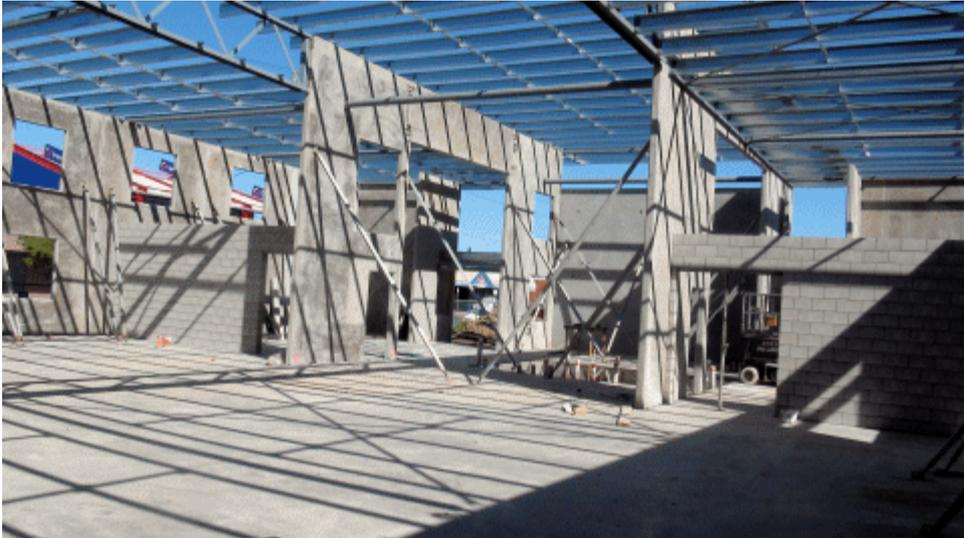
The auditorium, showing the rear block walls. Electrical conduits will be installed in these walls on Monday and the blocks continue up to roof level, then poured with concrete.
