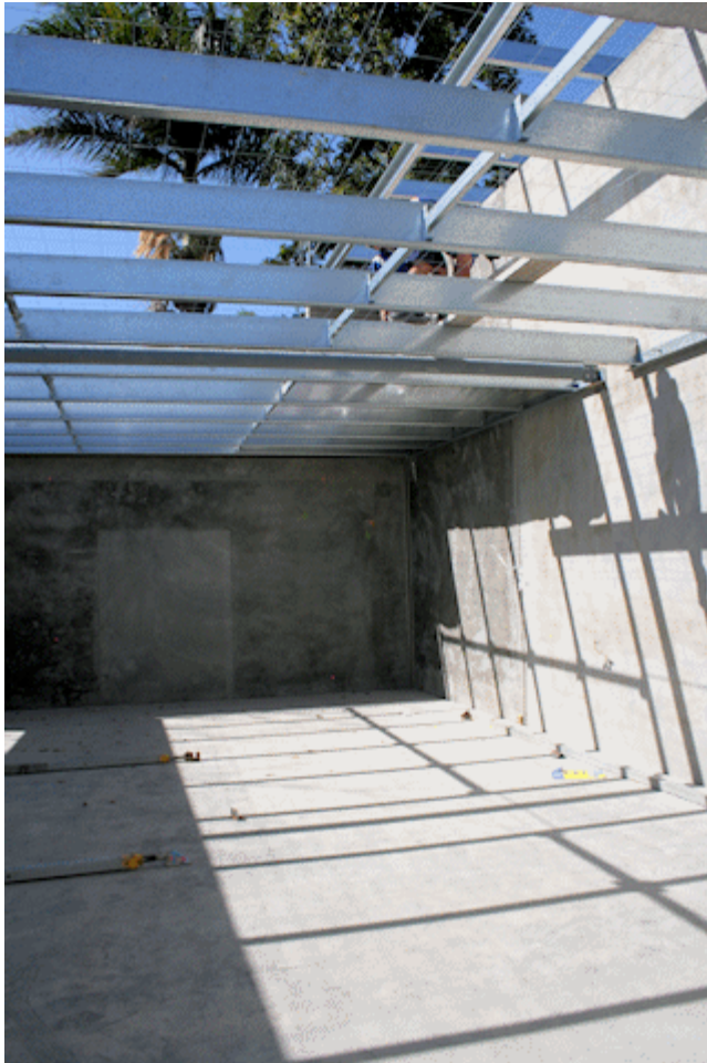
Sunday School / KFC with roof insulation and sheets being installed.
