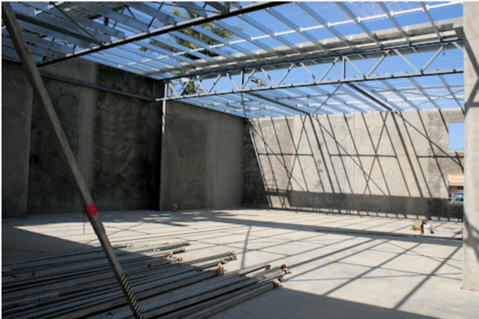
Auditorium with wall struts removed.
